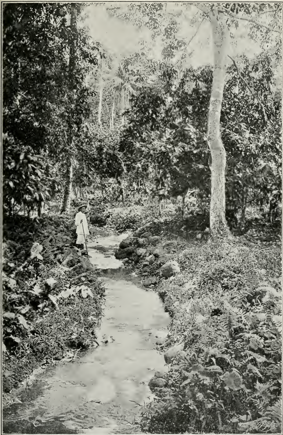
FIG. 40.—DRAINAGE WORKS ON RIGHT BANK OF PAPAGAIO RIVER, TERREIRO VELHO.
